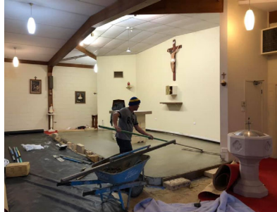
4. First level of concrete laid.
